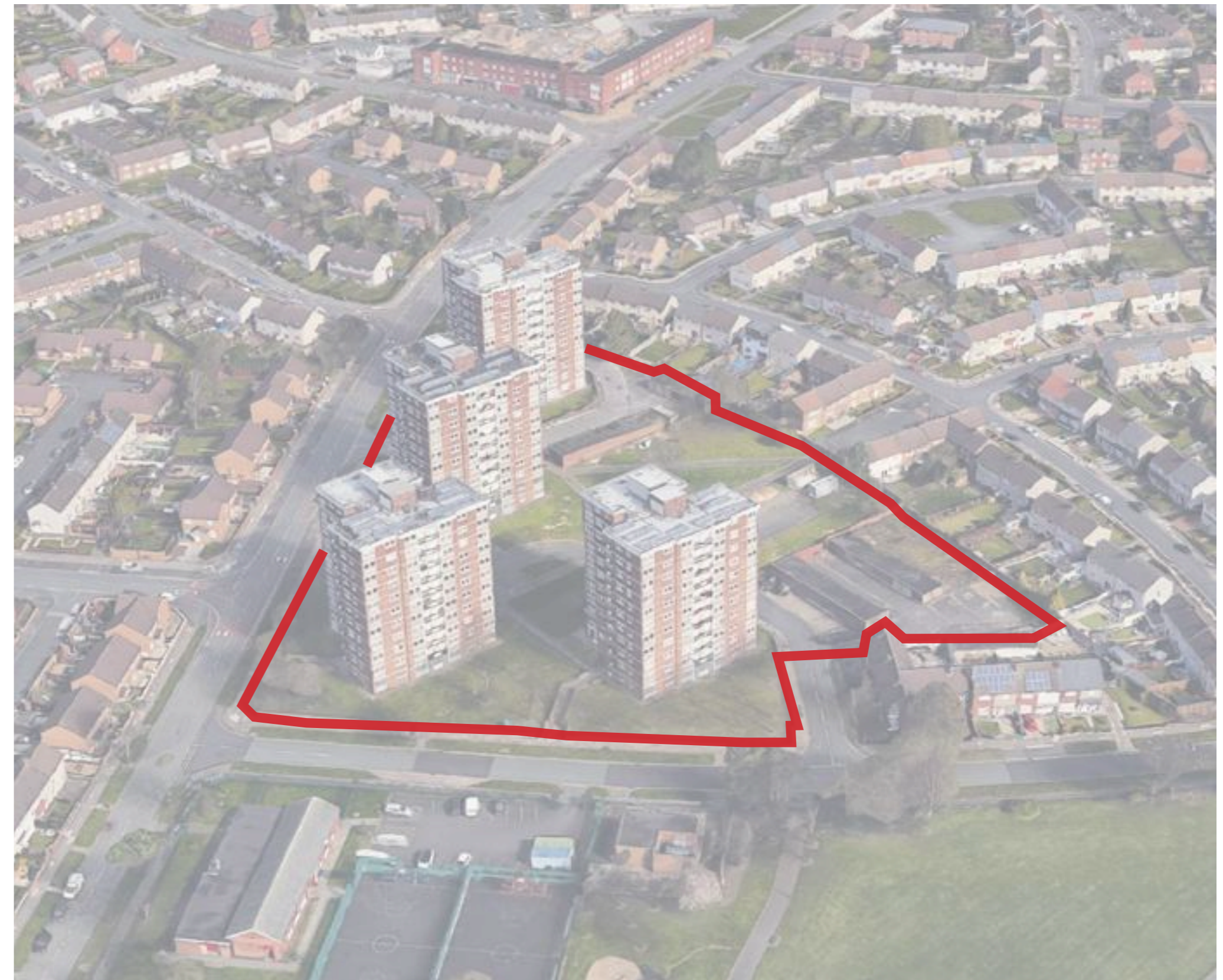
The existing site at Gaywood Green
